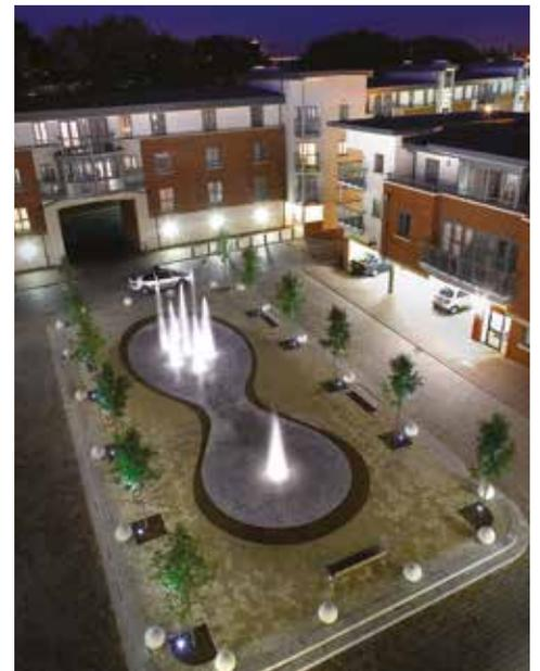
landscape architect and the landscape contractor enabled these issues to be overcome. During the works, Oak View suggested turning the alignment of the block that butted up to the curvy stainless steel edge through 90°. In this way a better relationship between the two could be achieved with precise neatly cut blocks. This was implemented to good effect.
